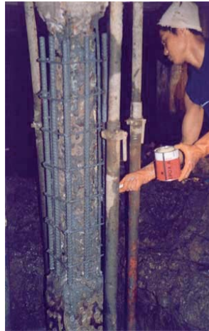
Application of Epoxy Bonding Agent
