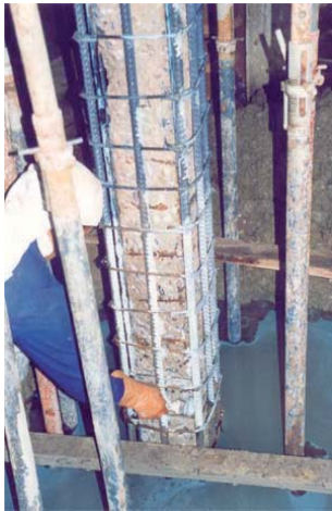
Two coats of Anti-Rust Protection
