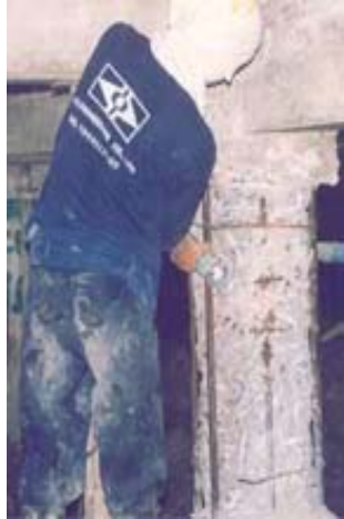
Remove rust on reinforcement steel
