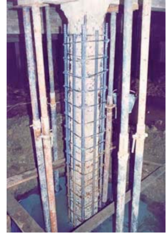
Column prepared and new reinforcement fixed for re - casting repair
