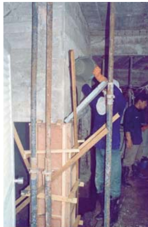
Repair with Non-shrink Grout
