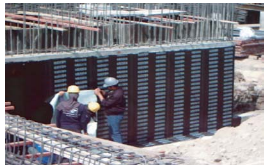
BASEMENT WALL APPLICATION
